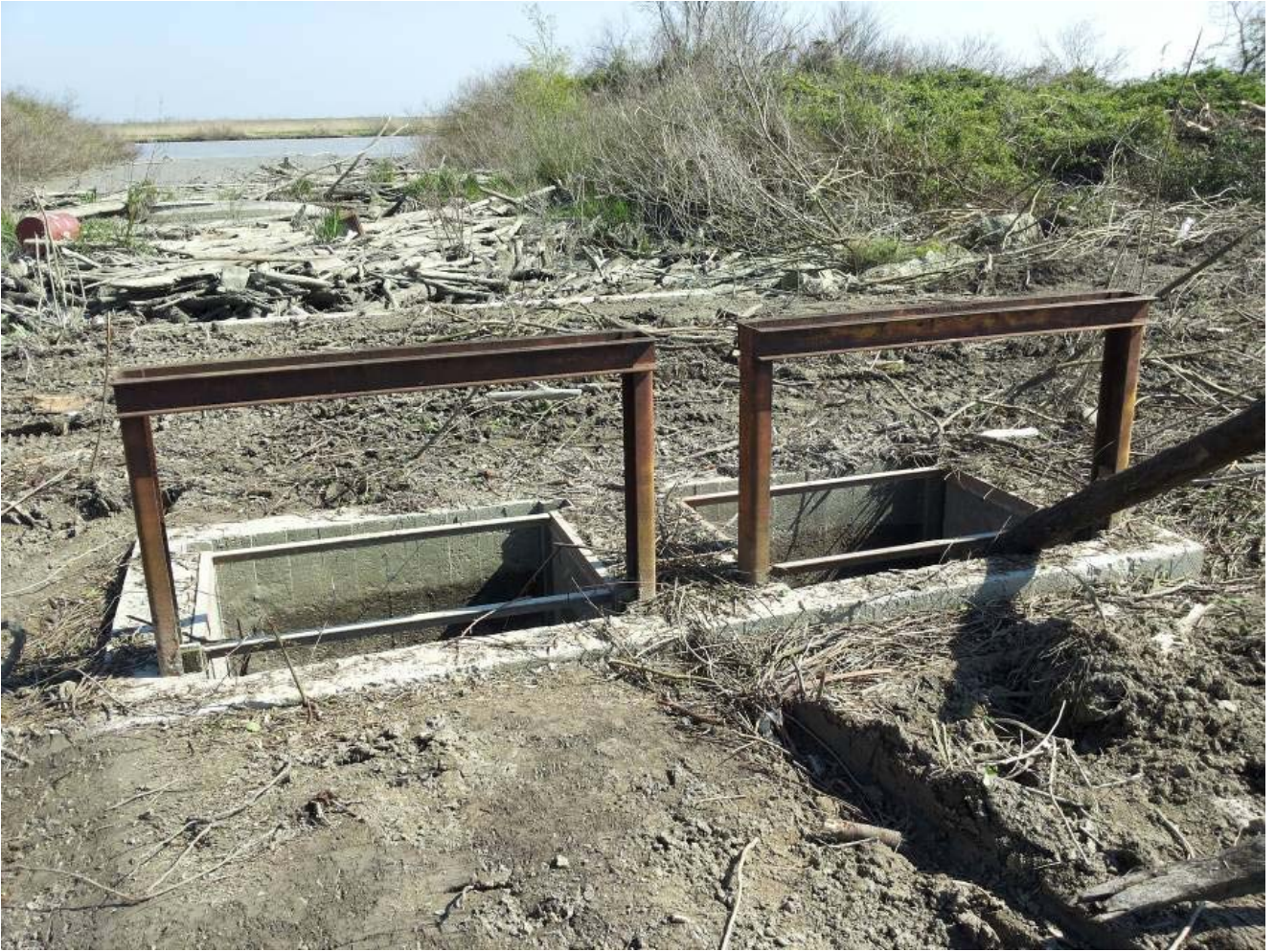
Pictures 1 and 2. The actual situation of the hydraulic structure
